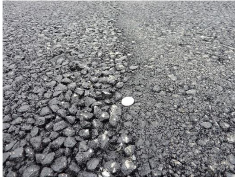
Figure 6. Area known as end-of-truck-load segregation (corresponds to the distance 1506 m in Figure 4).
