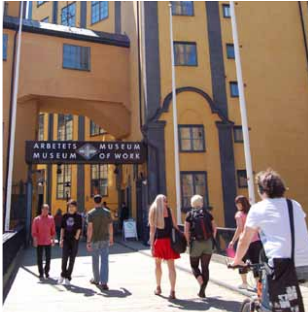
New life is breathed into the empty former textile industry premises, Norrköping.
