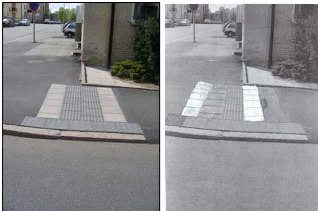
Picture 3 Suggestion for placing sinus slabs as a logical continuation of a natural guidance surface (right picture)
