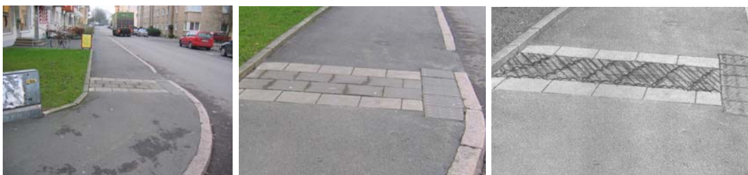
Picture 2 Suggestion for diagonally laid sinus slabs as guidance and/or direction indicator (right picture)
