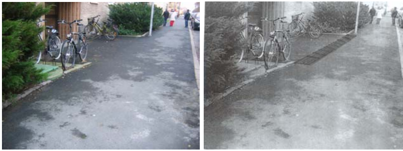
Picture 4 Suggestion for potential solution at entrance (right picture), longitudinal sinus slabs, width 35-40 cm. (Please observe that the pole at the end of the guidance surface must be removed).
