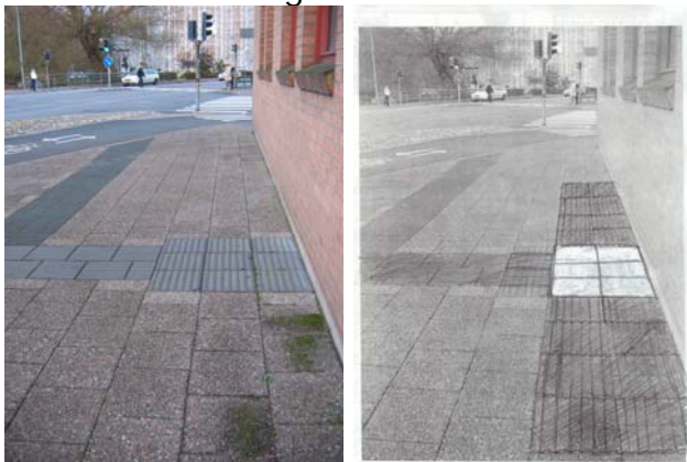
Picture 1 Suggestion for a potential solution: a decision surface in combination with a longitudinal sinus slab as a guidance surface (on the right)
