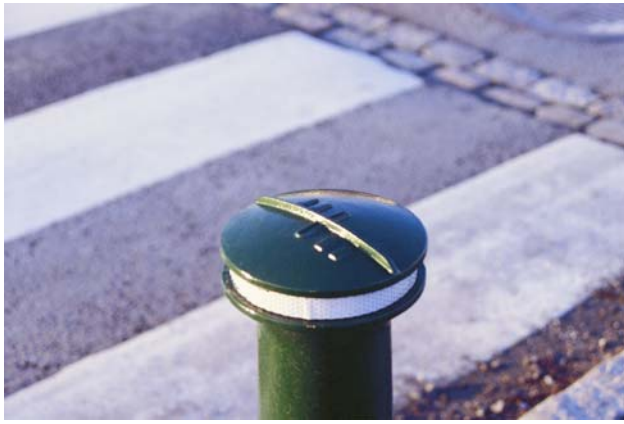
Picture 6 Bollard with map designed so it can be felt horizontally
